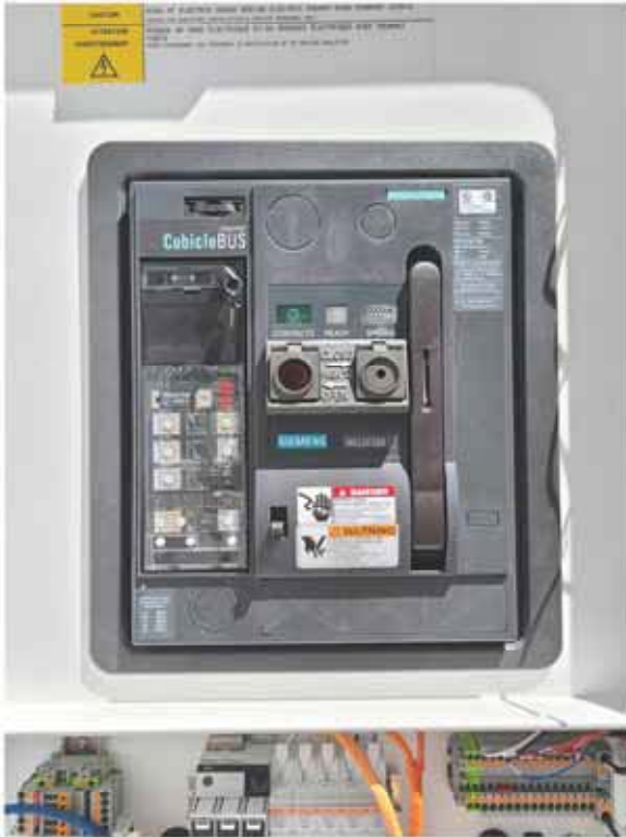
Figure 40. AC Circuit Breaker
