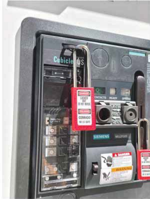
Figure 44. AC Circuit Breaker - With Additional Spring Charging Lock Out
