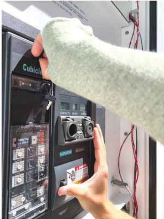
Figure 42. AC Circuit Breaker - Unlocking the Lock Ring
