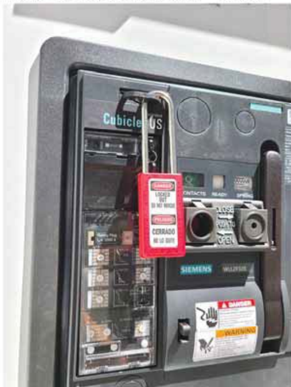
Figure 43. AC Circuit Breaker - Locked
